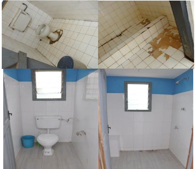
Before and after pictures of some of the renovations
